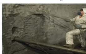
喷涂界面处理剂 Treatment agent on spray interface
