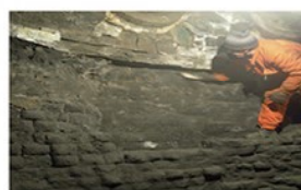
清理碳砖的氧化粉化层 The oxidative layer of carbon bricks cleaning up
