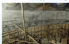
模具支设 Erection of molds
