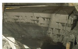
局部补砌碳砖 Carbon bricks supplementing
